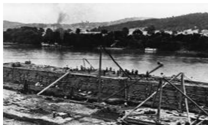
Mississippi River Improvement, 1890 (U.S. Army Corps of Engineers)
