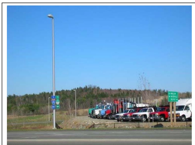
O'Connor GMC's truck lot at the eastern landing of the new Third Bridge.
